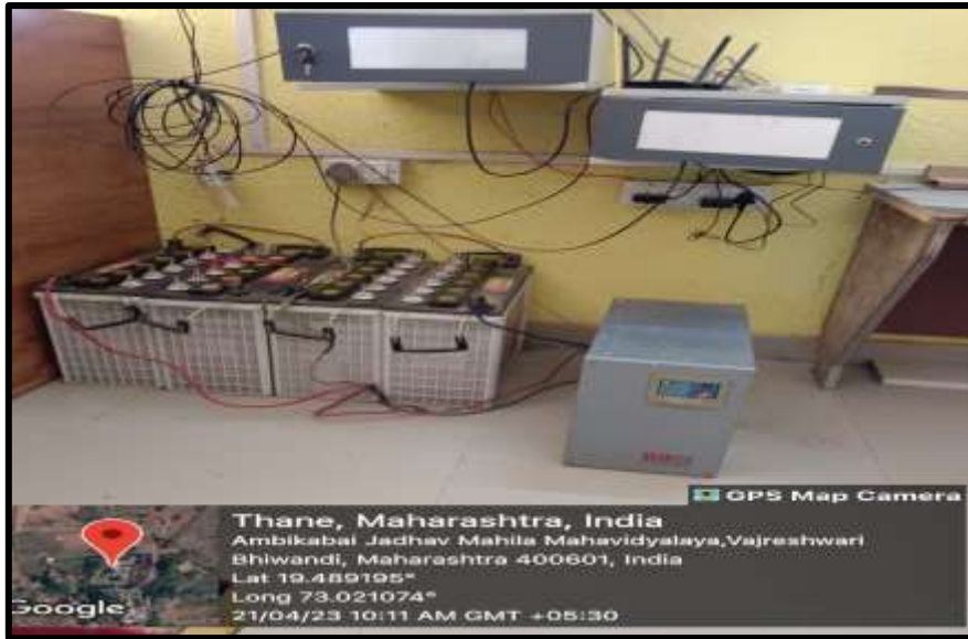
Figure 13- Main Building Wi-Fi Section
